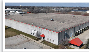
BROOKSHIRE SELECT SITES A TURNKEY APPROACH TO PROMOTING YOUR INDUSTRIAL SITE
